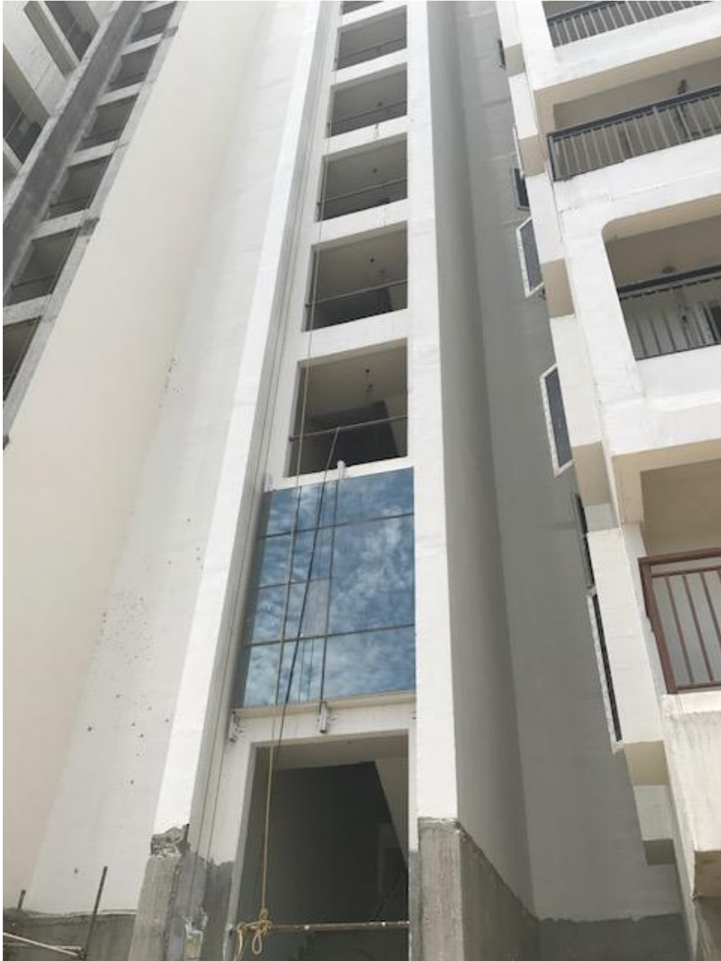
STAIRCASE GLAZING IN B BLOCK
