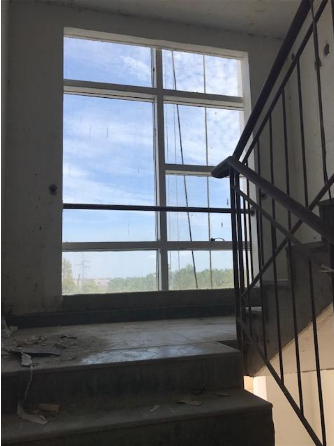
STAIRCASE GLAZING IN B BLOCK
