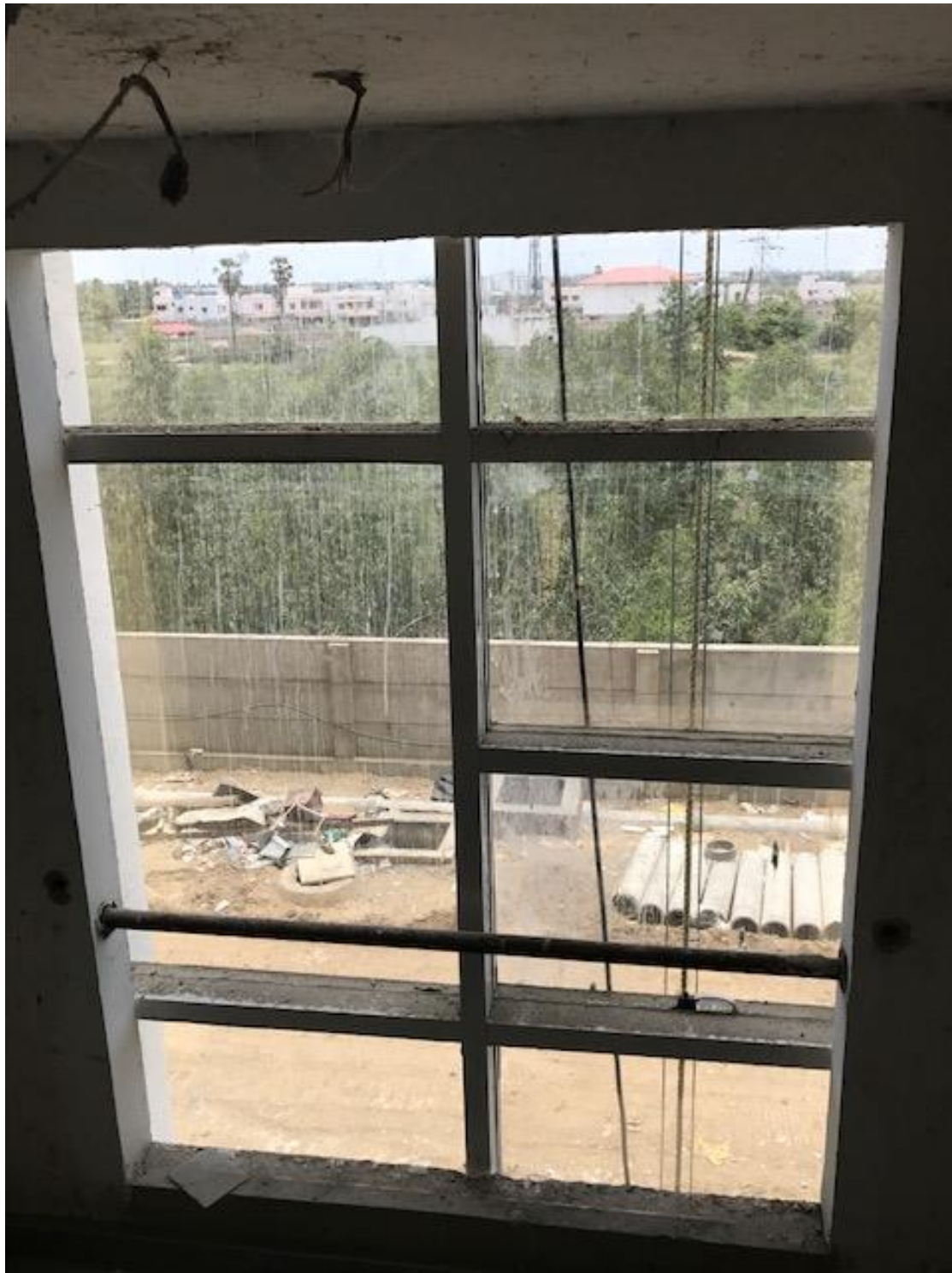
STAIRCASE GLAZING IN B BLOCK
